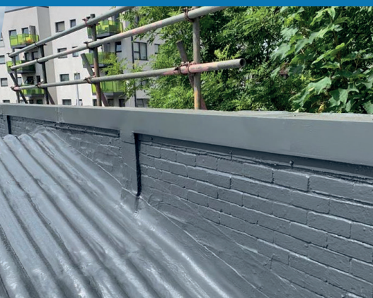
Coating Extended up Parapet Wall
