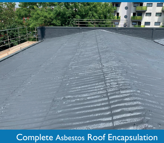
Coating Extended up Parapet Wall
