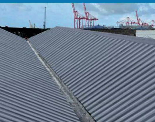
Complete Asbestos roof Encapsulation
